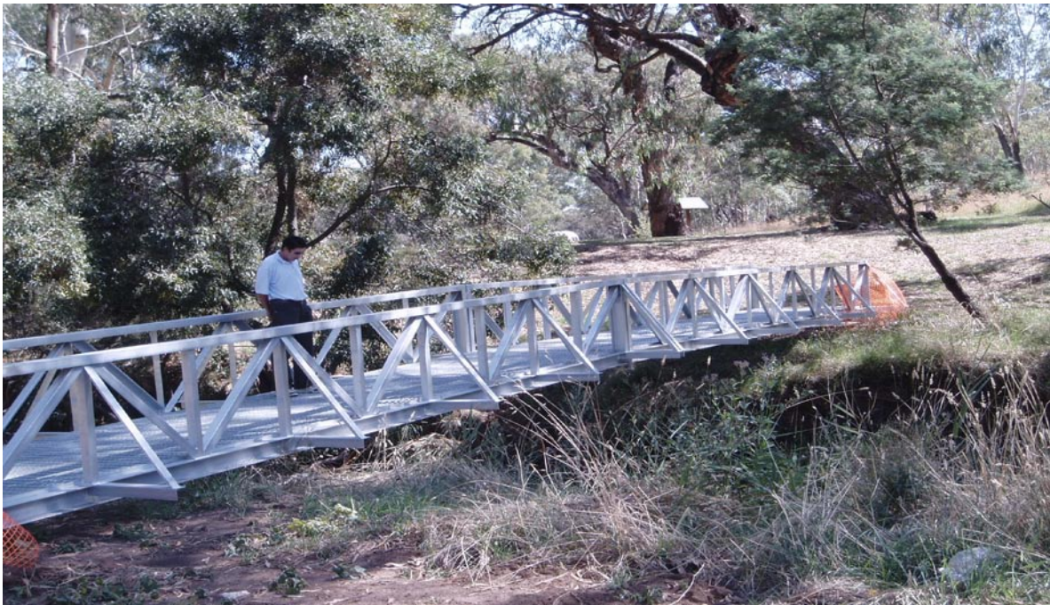
New footbridge at Borenore Caves
